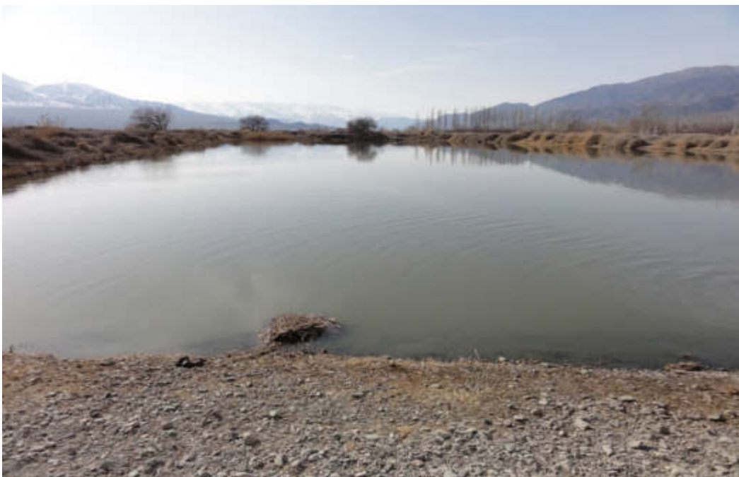
Photo 4. Balykchy WWTP. Existing pond Karakol Wastewater Treatment Plant
