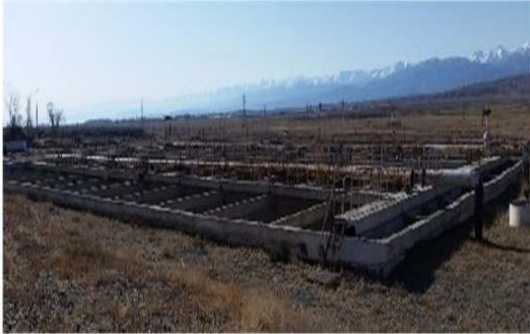
Photo 1. Balykchy WWTP. Existing aeration tank
