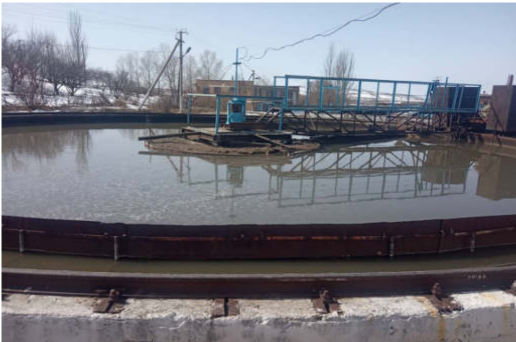
Photo 7. Karakol WWTP. Pre-sedimentation Tank
