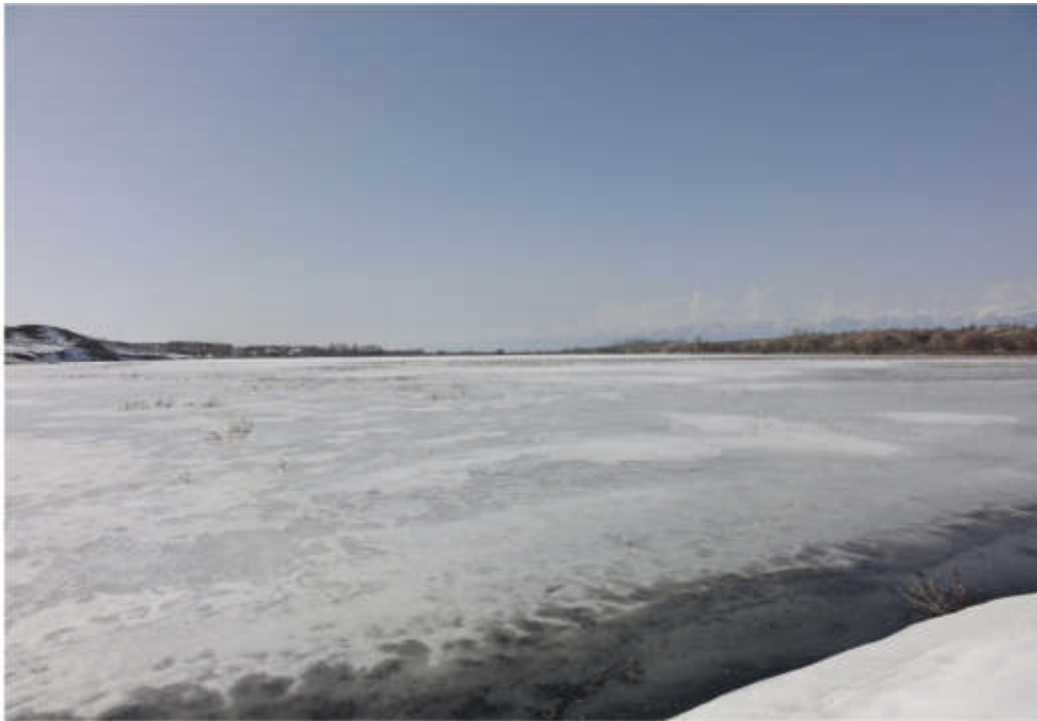
Photo 6. Karakol WWTP. Seasonal Runoff Pond
