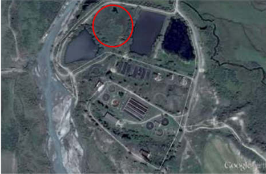
Figure 13 Existing WWTP of Karakol and the location of the Central Asian frog
