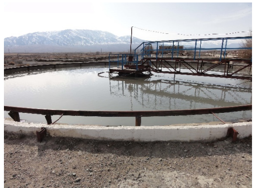
Condition of WWTP Balykchy
