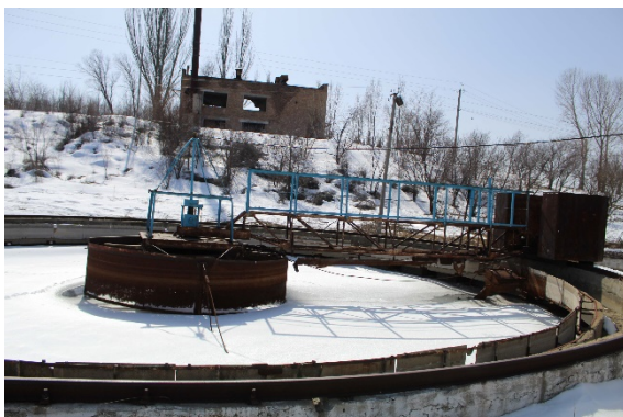
Condition of WWTP Karakol
