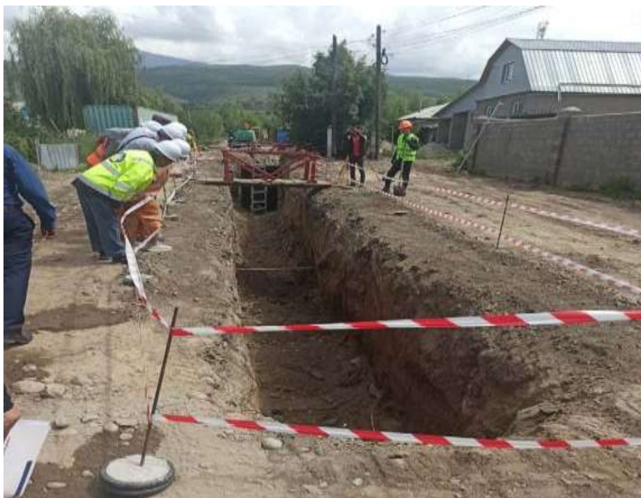
Figure 2-7 Construction site of Minur Ltd.
