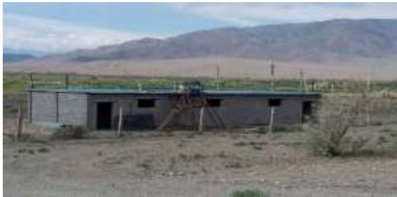
Figure 2-9 Temporary structures at WWTP
