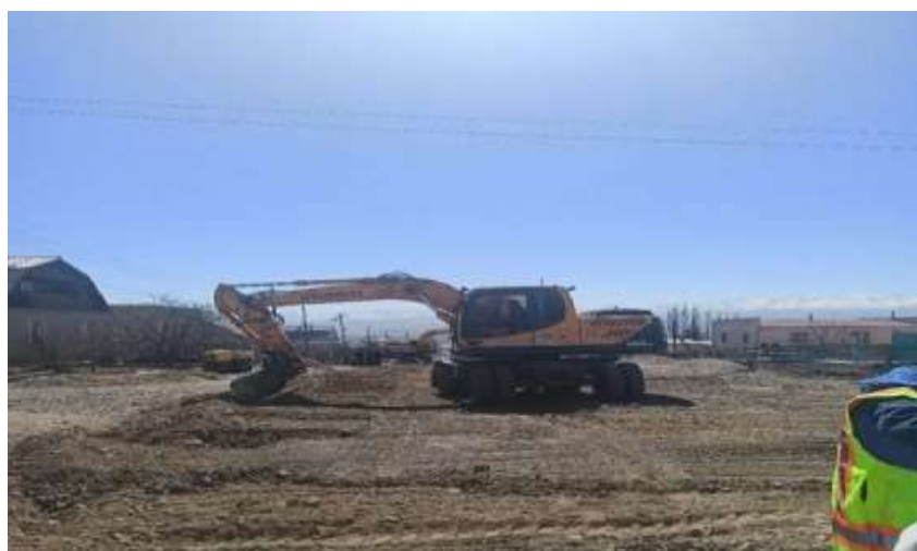
Figure 2-6 Construction site of Profit Express Ltd.
