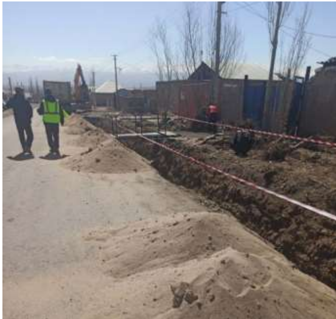
Figure 2-5 Construction site of Impulse Osh Ltd.
