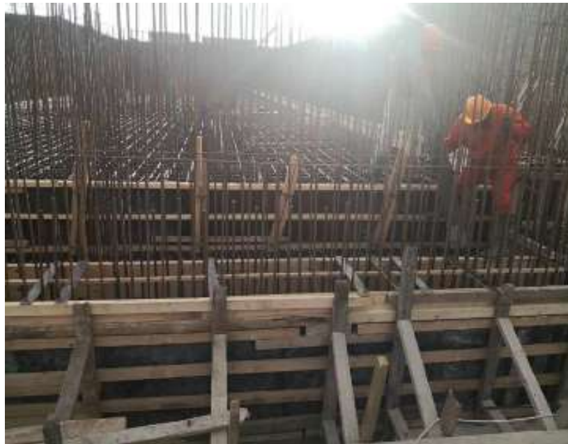
Figure 2-12 Construction site of WWTP
