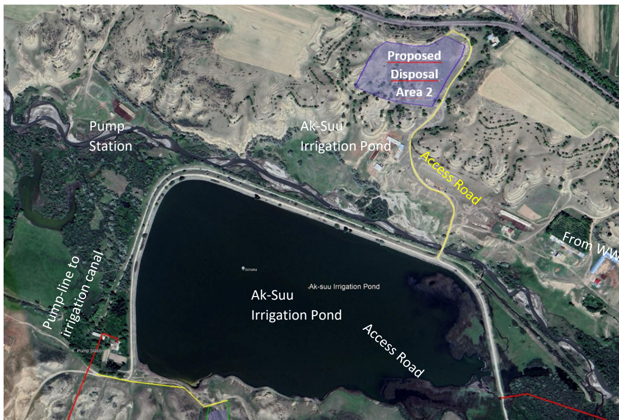
Figure 5-5. General Layout of Alternative-2 Site for the storage area in BSR of AKSU DDWR
