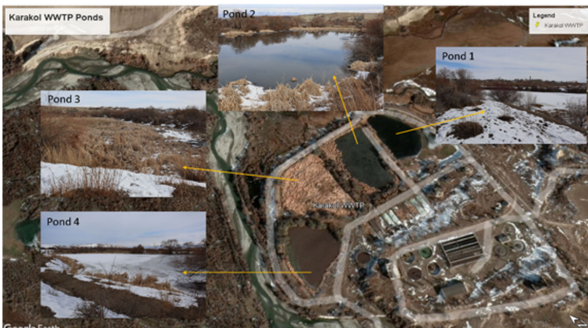
Figure 2-2. The overview of Karakol wastewater stabilization ponds
