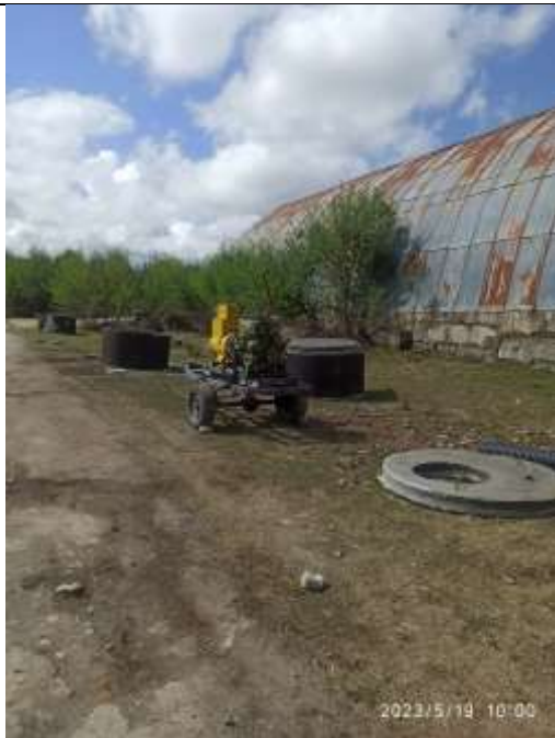
Construction site has to be demarcated using proper barricading
