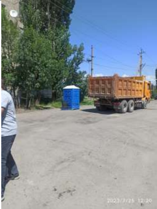
Mobile toilet facility is provided in the site
