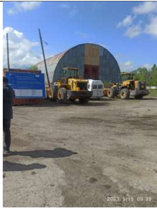
Construction vehicles are parked within the construction camp
