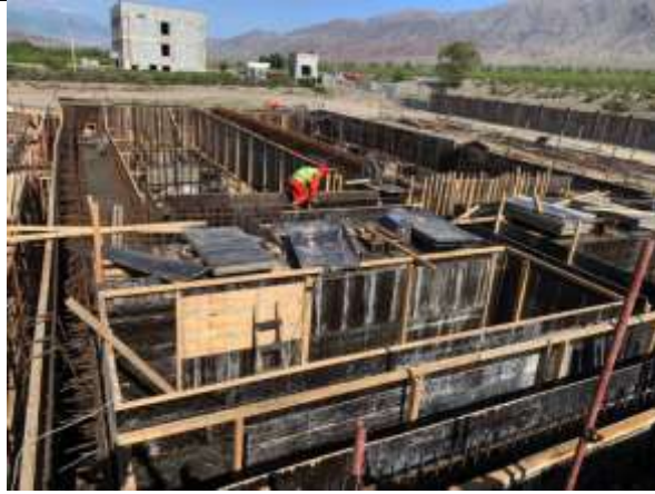
Formwork Installation Sedimentation Tank
