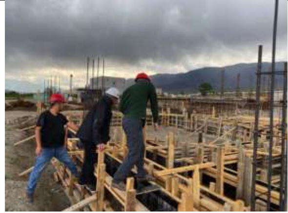
Boiler – Blower Room foundation formwork
