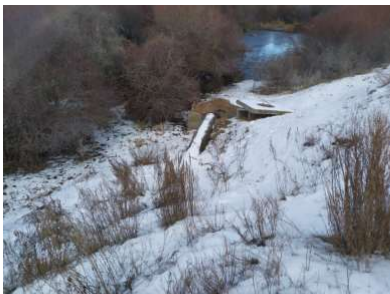
Figure 3-4: Karakol River Crossing
