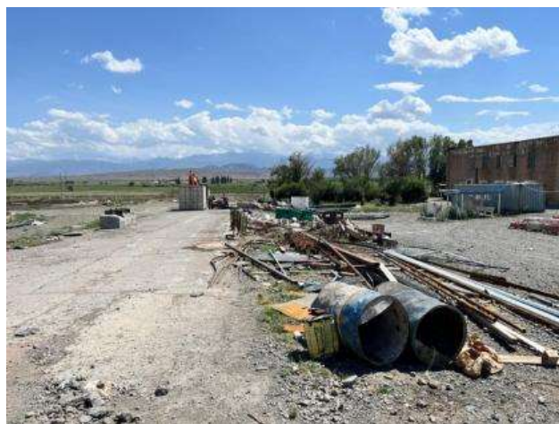
Balykchy WWTP - Construction waste are not stored as per the management measures given in the SSEMP (June 2024)
