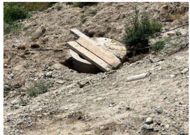
Septic tank cover is partially closed, which will lead to mosquito breeding
