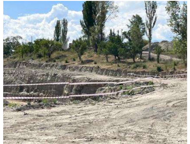
Hard barricading should have been provided for the excavated areas
