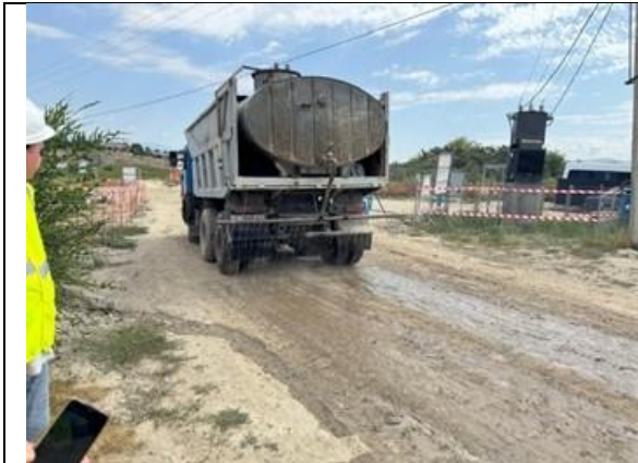
Dust suppression measures have been adopted
