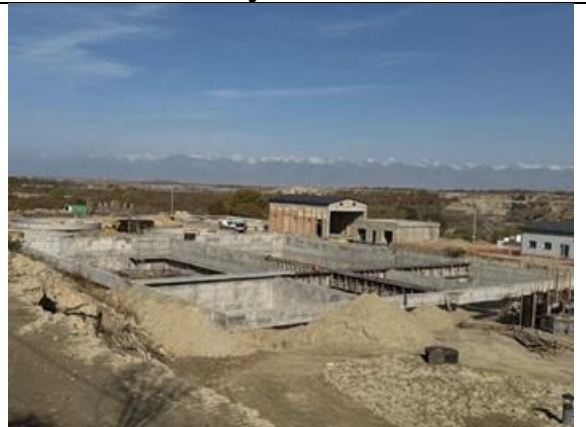
View of the WWTP site
