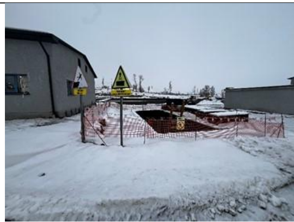
Barricading has been provided for deep excavated areas
