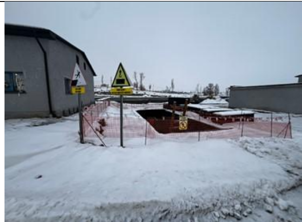
Multilingual hazard signage and Red mesh fencing installed
