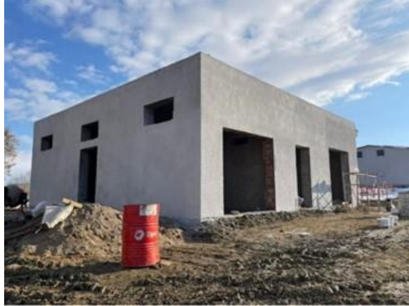
Transformer Building - Appropriate scaffolding arrangements are observed
