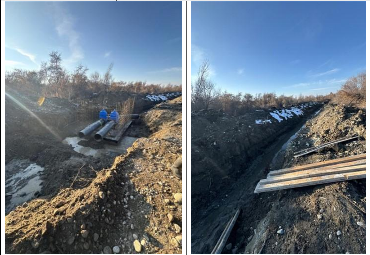
Pipelaying works are in progress on Alybakova and Lenin Streets
