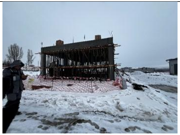
Barricading has been provided
