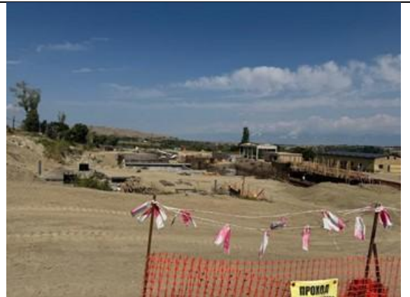
Barricading has been provided along with the safety information board
