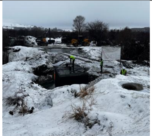
Site signage installed and Workers in high visibility jackets and helmets
