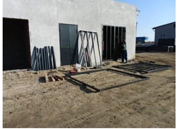
Worker in safety vest (PPE's) and Organized material staging
