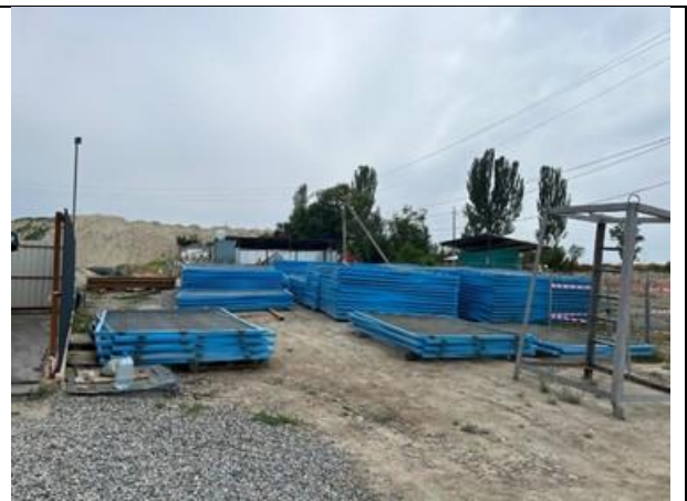
Shuttering materials are stored in designated areas
