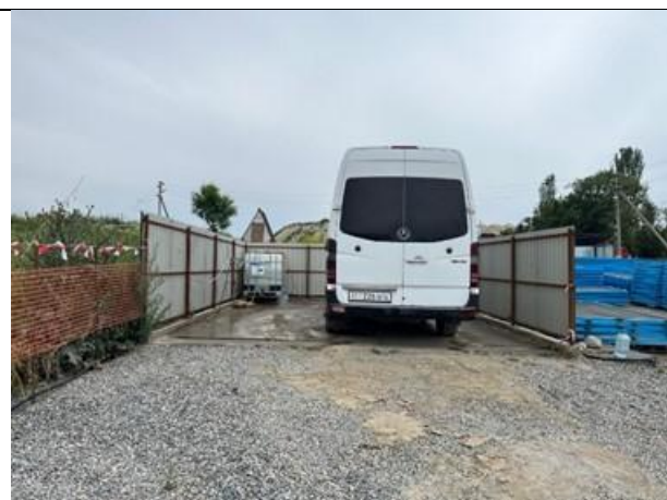
Construction vehicle wash area provided
