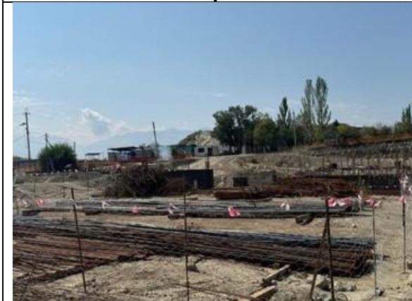
Construction materials are stored in the demarcated area
