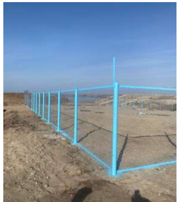
Sewerage Receiving Tank Site (50 m 3 ) with Backfilling and Fencing
