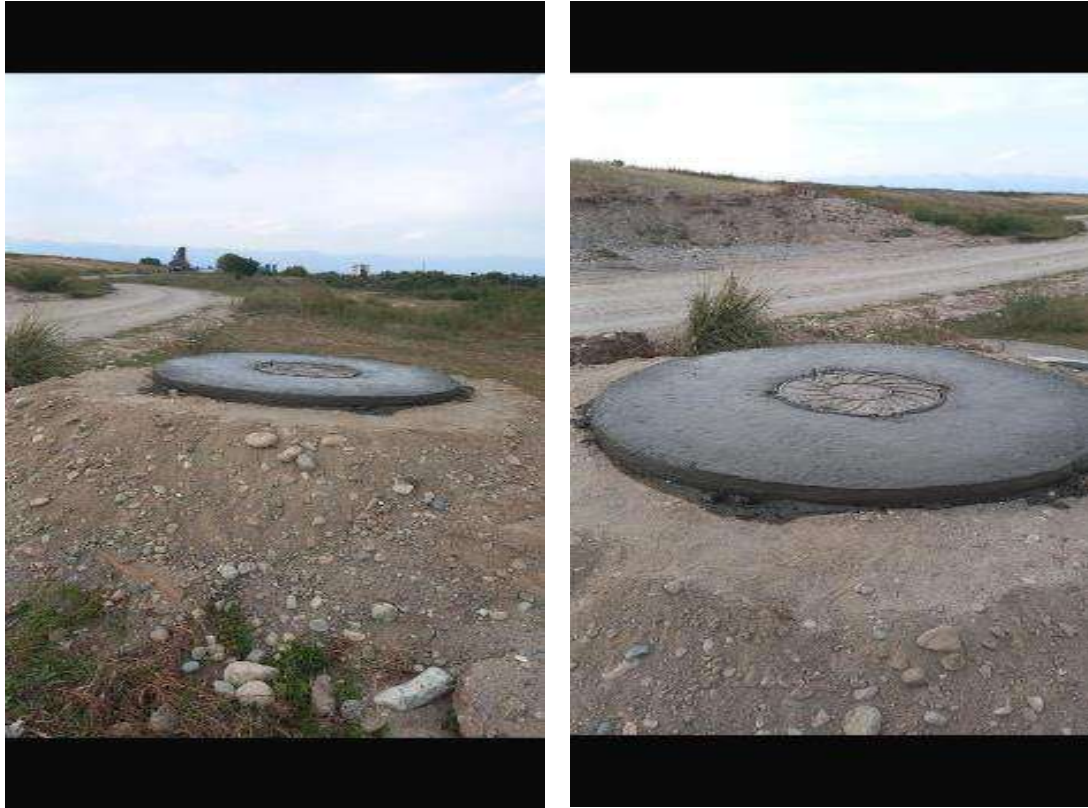
Manhole cover after rehabilitation
